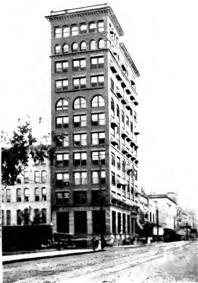
THE D. T. PORTER BUILDING
